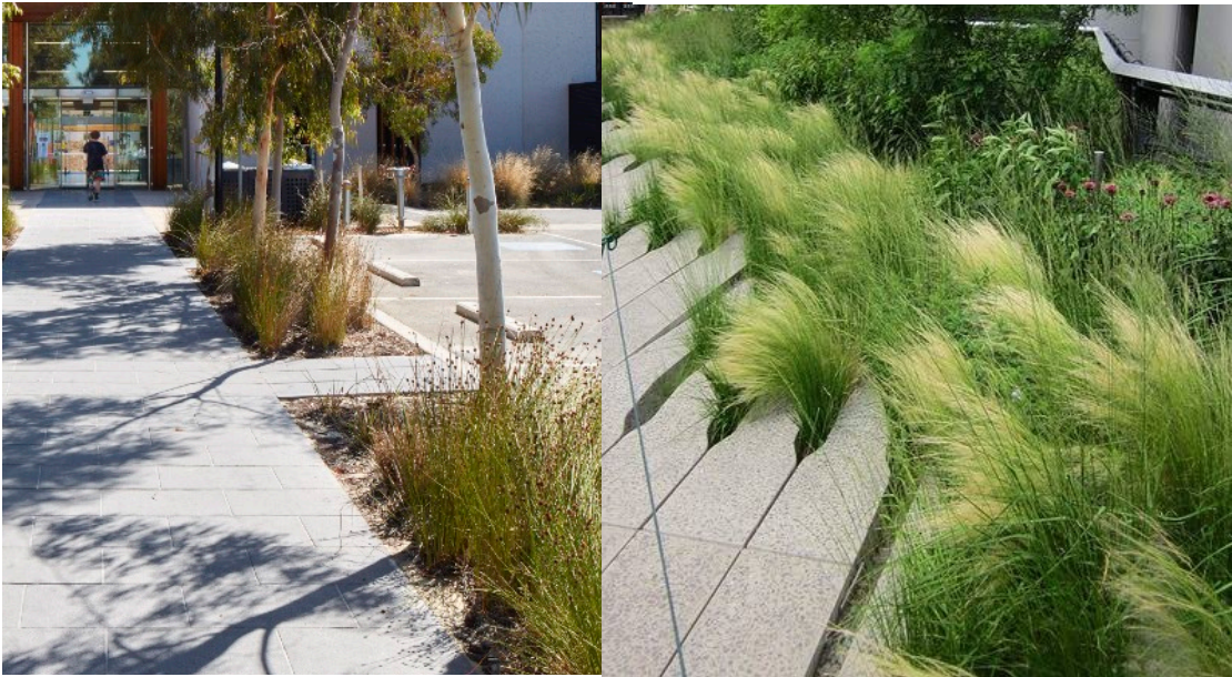
Grading to Tree Pits / Permeable paving Integrated permeable paving and planting of littoral and native grasses.
